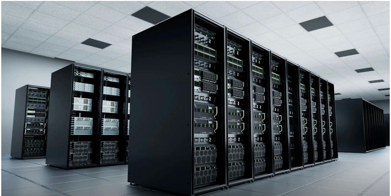
Grace Hopper Data Center Racks: "Data Center Frontier"
